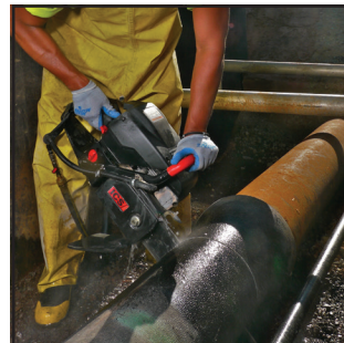
Safer to cut ductile iron
